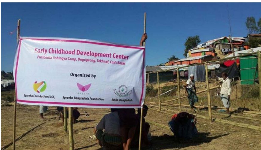
Spreeha Early Childhood Development Center construction
